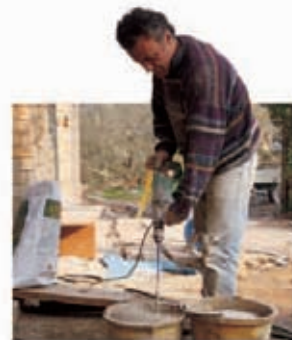
建築屋 kenchiku-ya construction worker
